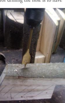
**6.** Before you nail it all back together just drill some pilot holes (about 25% less in diameter than the nail itself), which should stop any splits occurring. Also, make a mark directly opposite the entrance hole on the back wall and drill a clearance hole for a screw. You should then be able to access the screw through the entrance hole to fix the box to a suitable tree or post. Put the screw in NOW – it is much easier than when you have put the lid on!
